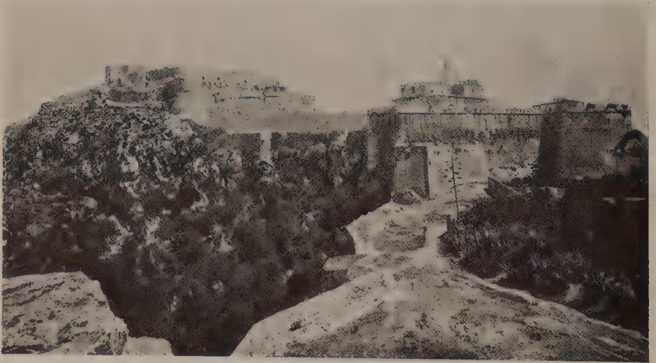
MILAZZO CASTLE, SHOWING OUTER WORKS AND KEEP.
